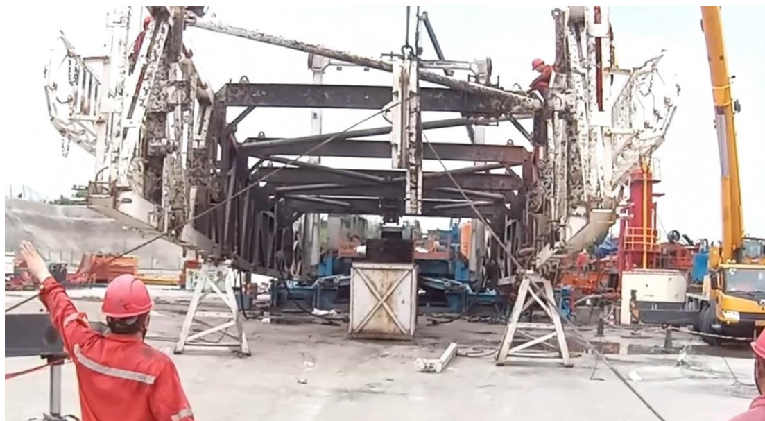
Figure 3.1 Actual scene of derrick disassembly and assembly
