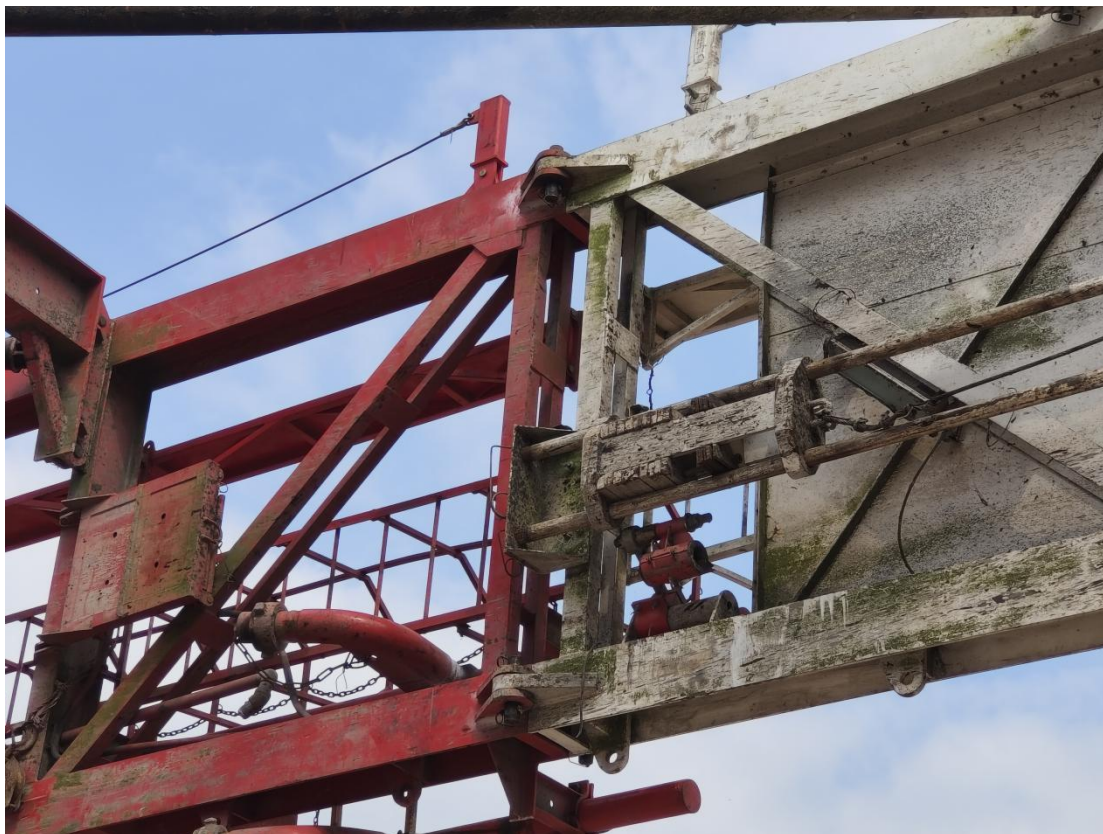
Figure 4.6 Working position of pins at the derrick disassembly and assembly site
