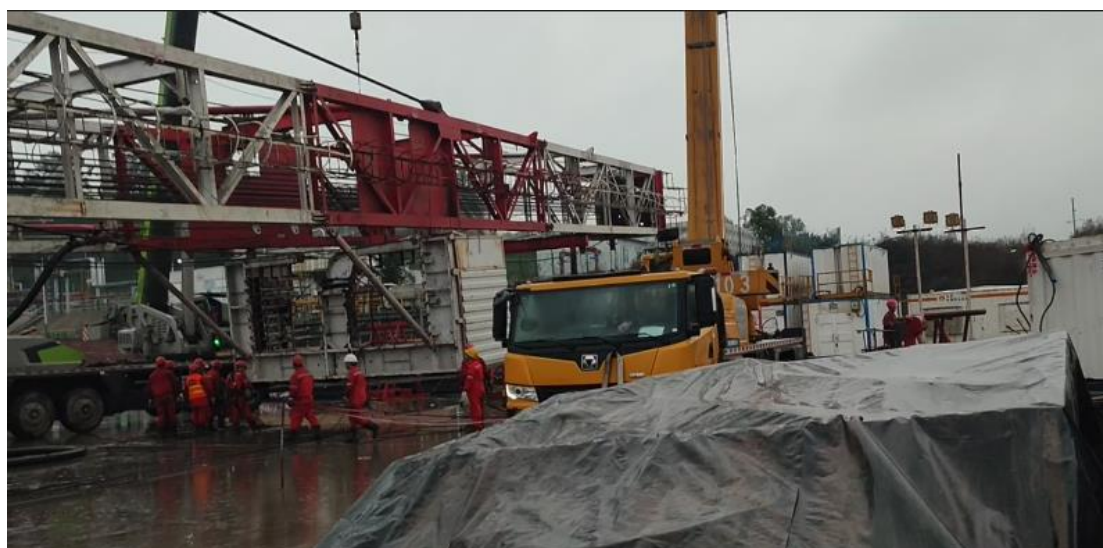
Figure 3.3 Work site in heavy rain
